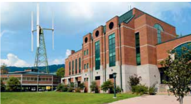
Commercial operation: Reduction of electric bills by providing one's facilities with one's own distributed source of power e.g. waste water plants, desalination plants
